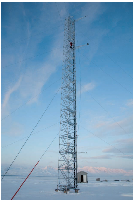
Picture of the 34 m Climatic change tower
