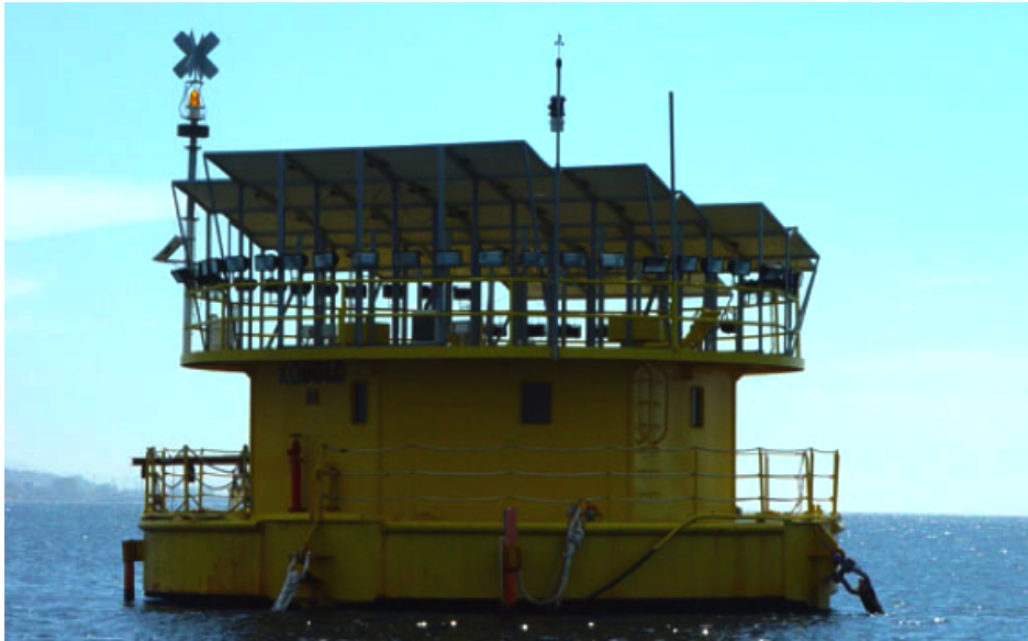
Figure 1: The ENERMAR-Kobold platform in the Straits of Messina: a prototype built to extract energy from the marine current flow (patented in 1998 and owned by Ponte di Archimede International).
