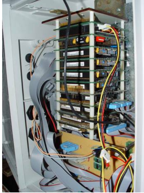
Figure 4: The watertight box containing the control computer; the vertical bottom board hosts the XBT probe interface.
